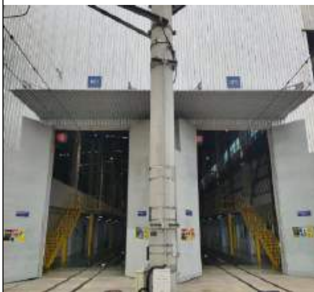
Inspection Shed / Gedung Inspeksi
